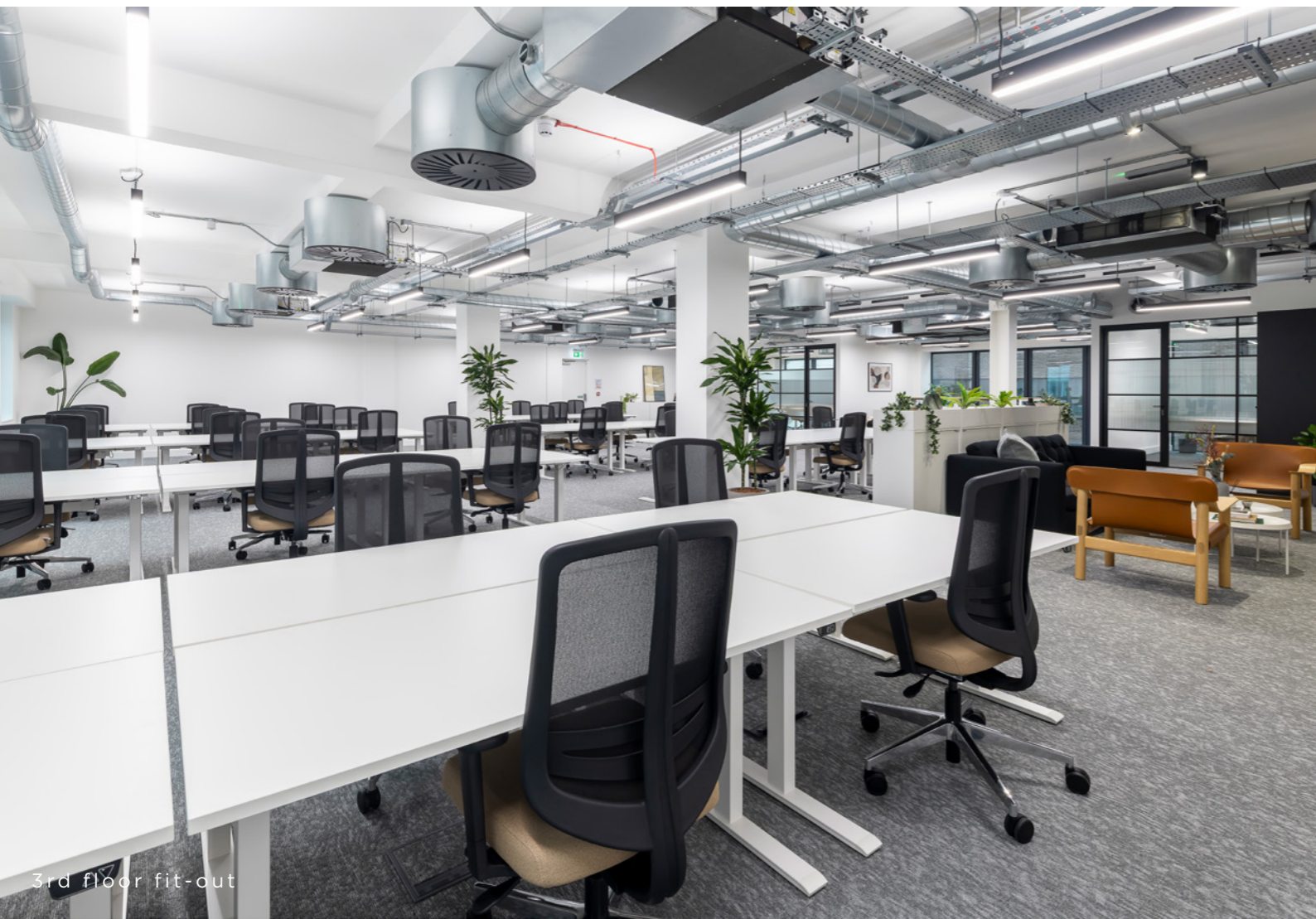
3rd floor fit-out
